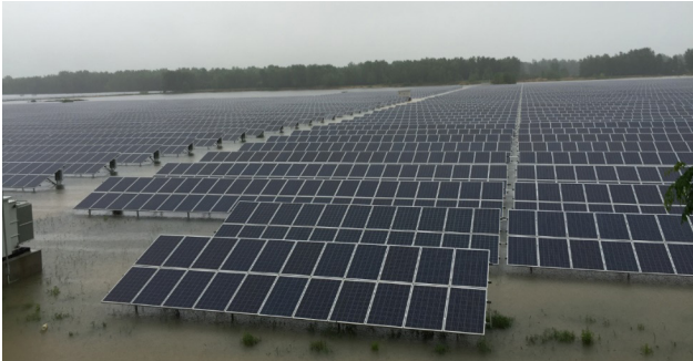
图1 光伏电站在麻城“7.1”暴雨中受损 Fig. 1 Flood disaster of the PV power station
